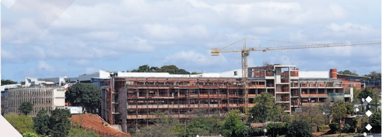
Almost complete! The new Engineering faculty block is taking shape
