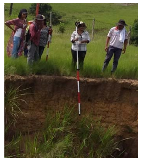
Students surveying the stream bank on which the foot bridge was to be constructed
